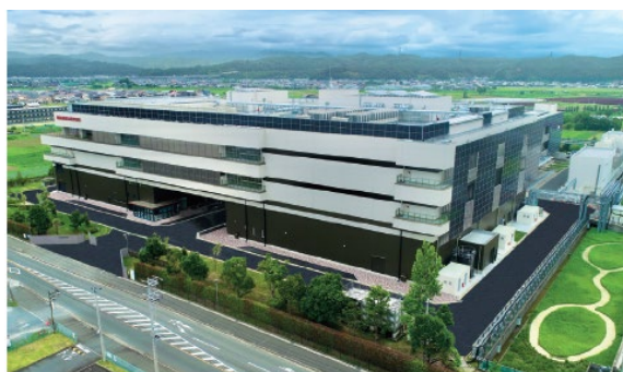
▲ Exterior view of new Toyooka Factory building (Electron Tube Segment)
